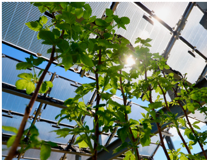
Fig.80 - In 2021, a first larger agro-photovoltaic plant was put into operation in Switzerland. The technology was developed by the start-up Insolight and is based on translucent solar modules, where the transparency can be varied using optical micro-tracking. The installation covers 165 m 2 on a raspberry production farm. Other participants in this pilot project, supported by the SFOE, are Romande Energie as utility and Agroscope, the national centre of excellence for agricultural research (Image source: Insolight SA)
