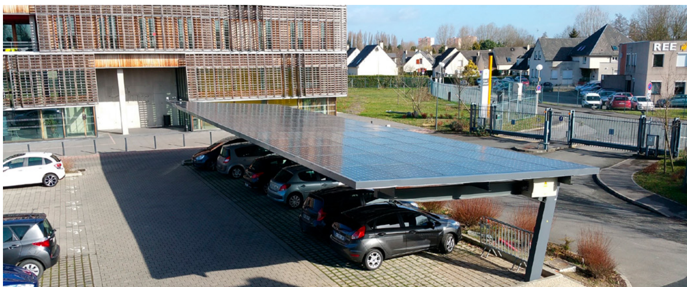
Fig.29 - PV-powered electric vehicles charging station based on microgrid on parking in Université de Technologie de Compiègne (UTC), France PV-powered charging station, with around 30 kWp PV integrated, 18 kWh stationary storage, and grid connection, was developed under the UTC project in 2017/2019. Since then, this charging station has functioned as a demonstration site for power flow optimization, power control, and for identifying preliminary requirements and feasibility conditions.
