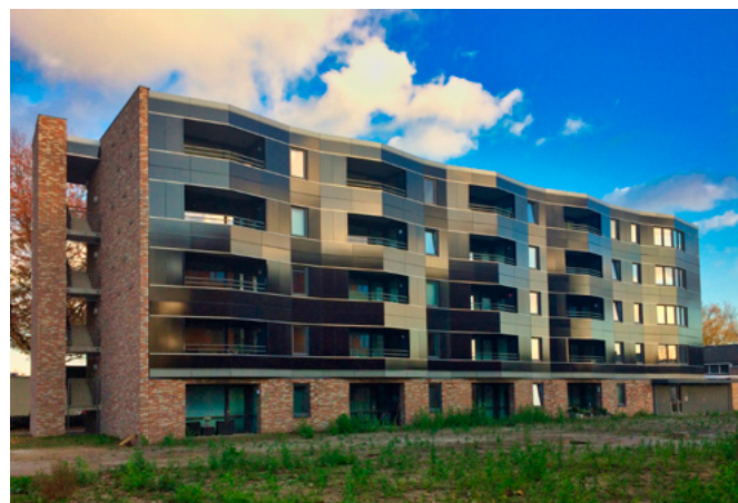
Fig.21 - Social housing apartment with BIPV facade, Best (NL) © BEAR-iD
