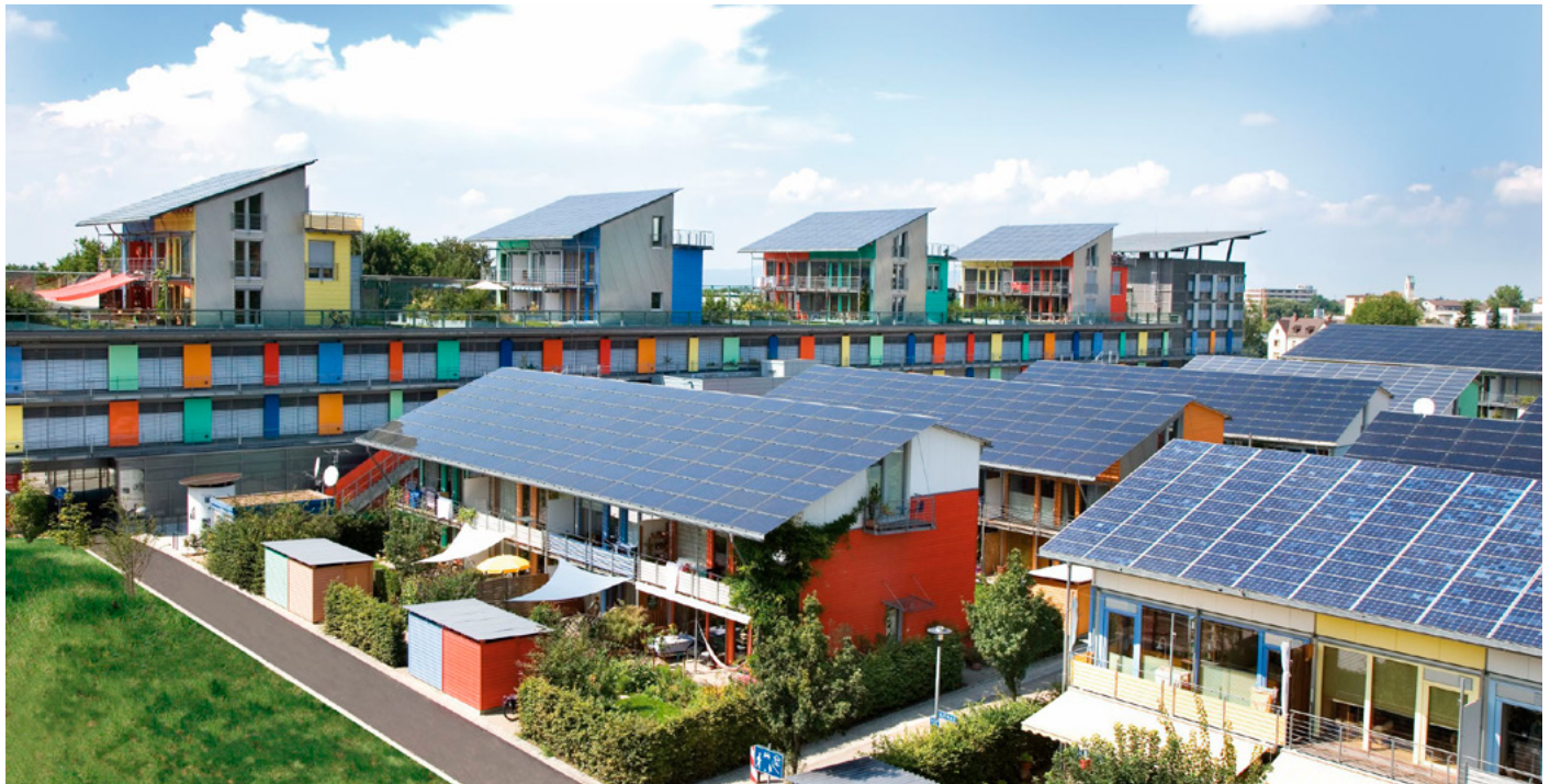
Fig.15 - Decentral Renewable Energy Systems like these local PV-roof installations at Solar-Siedlung Vauban, Freiburg have to support the stability of the energy network with ancillary services in the future. IEA PVPS Task14 presents solutions from IEA PVPS member countries on (smart) grid integration for a future 100 % RES based power system. (copyright Rolf Disch SolarArchitektur info@rolfdisch.de )
