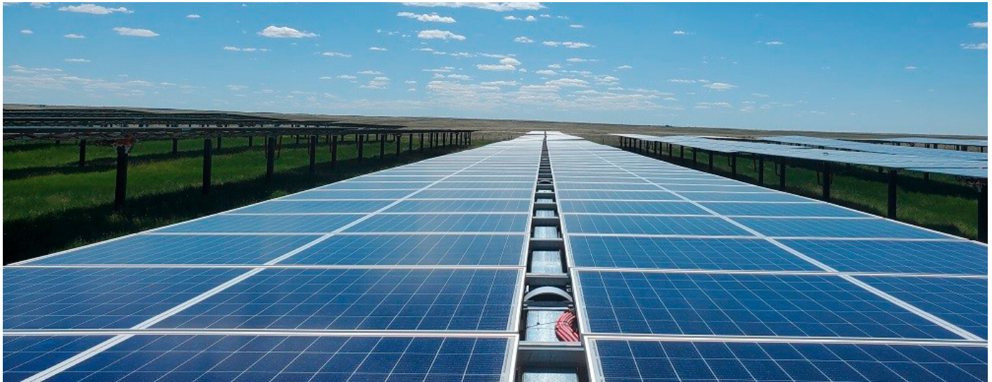
Fig.43 - Suffield, Alberta, 23 MW PV array consisting of bifacial modules and single-axis trackers. Photo credit: Matt Schuett (BluEarth Renewables).
