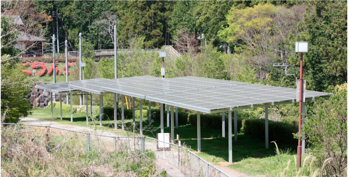
Fig.60 - PV system for regional microgrid at Odawara Kodomo no Mori Park Wanpaku Land in Odawara City, Kanagawa Prefecture, Generation capacity: 50 kW, c-Si PV modules: Kyocera, ©RTS Corporation
