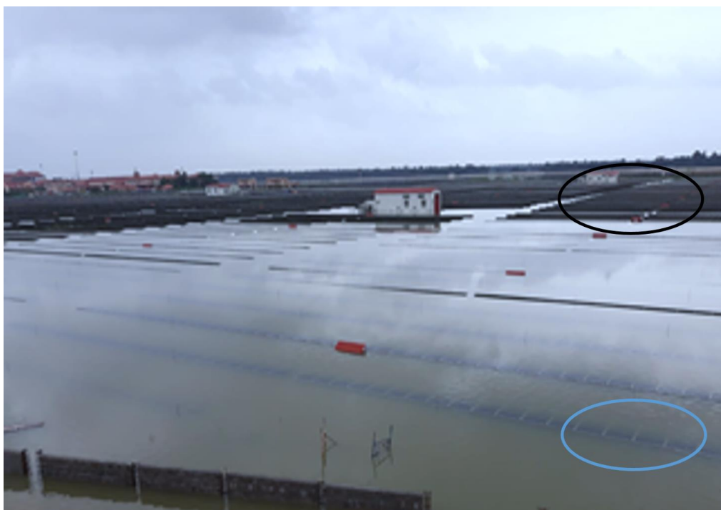
Figure 33: Partially submerged PV plant showing strings fully submerged in water (in blue circle) and those that are above water (in black circle).
