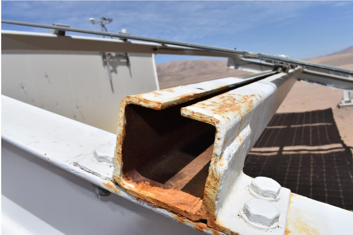
Figure 28: Rusty mounting structure in a PV power plant located in the Atacama Desert. This mounting structure has been in operation for about one year.
