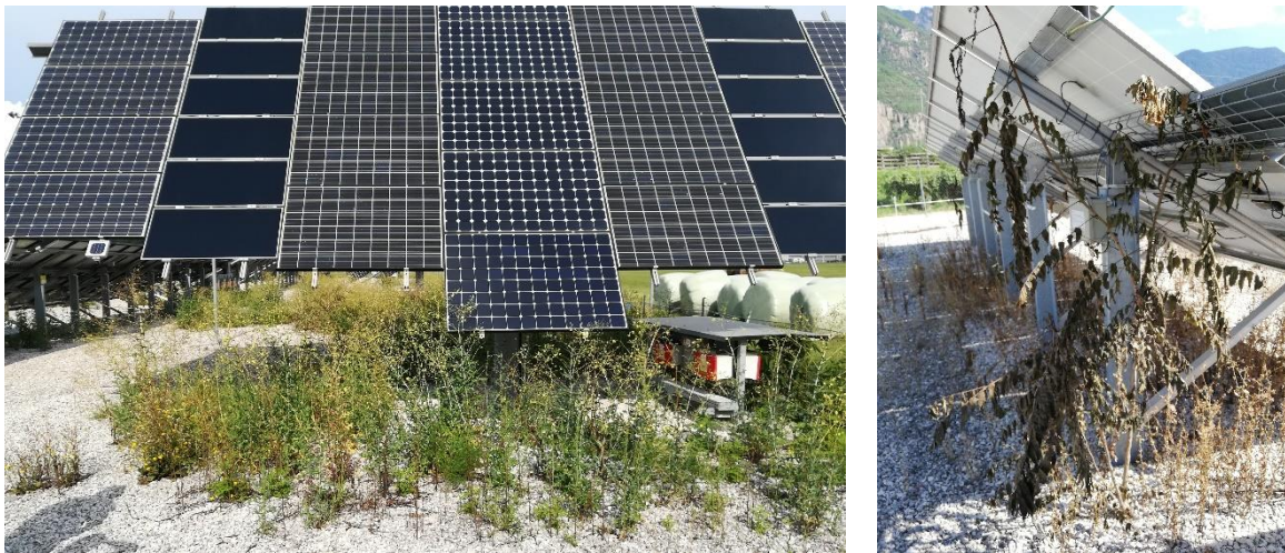
Figure 11: Growing bush in front of a tracker (left) and underneath an array (right) [Eurac Research].
