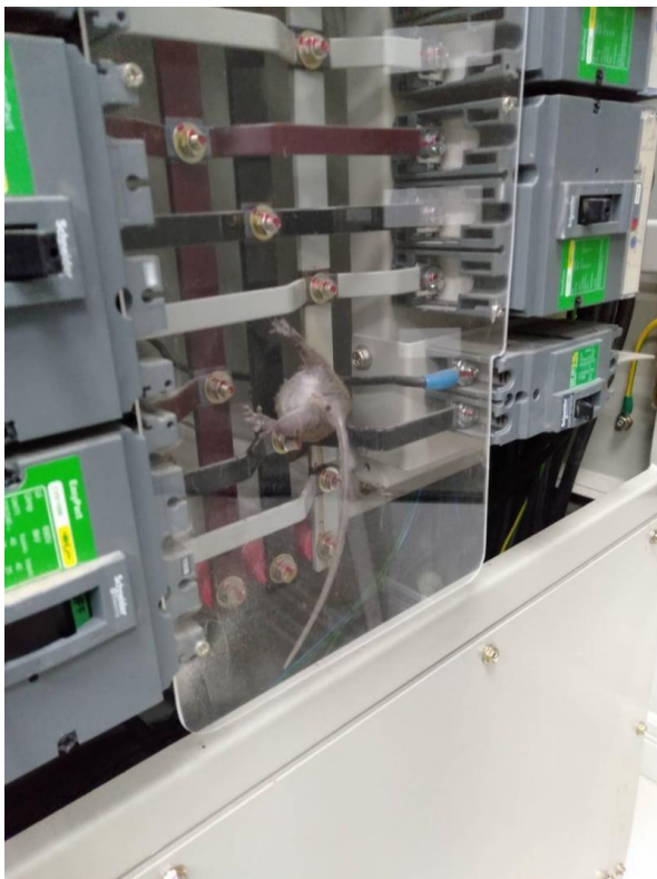
Figure 30: Impact by wildlife on PV components, such as a rat in the main distribution box (left) and termites around the DC cable under the PV module (right).
