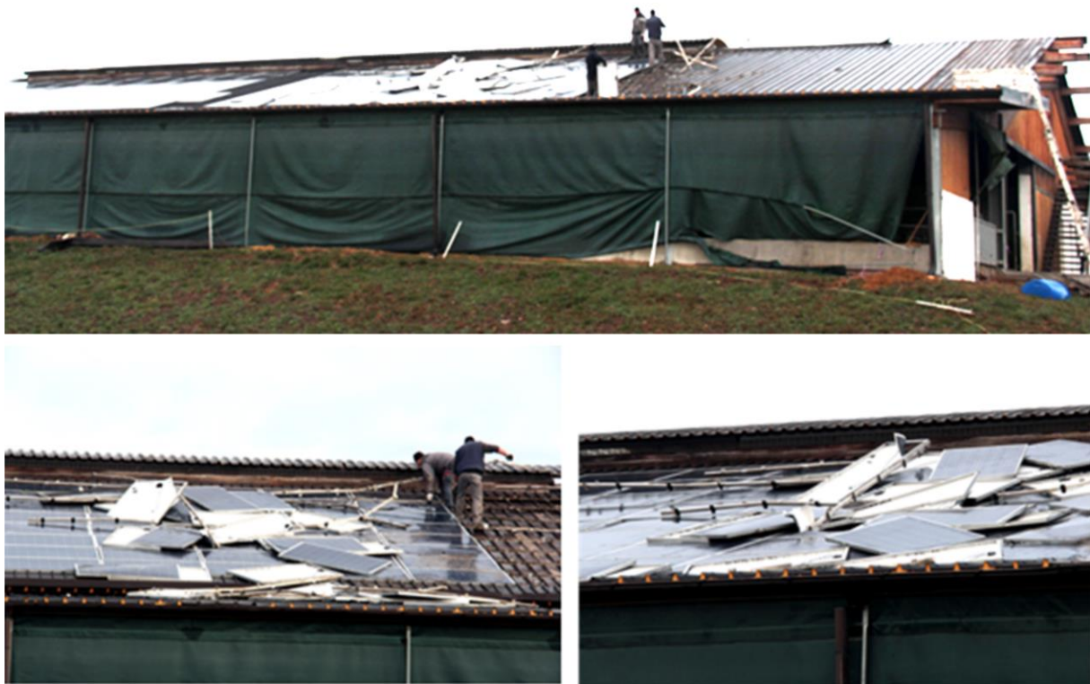
Figure 44: PV System status after a windstorm in Baselga di Piné, Italy. Source: Dino Loriatti.
