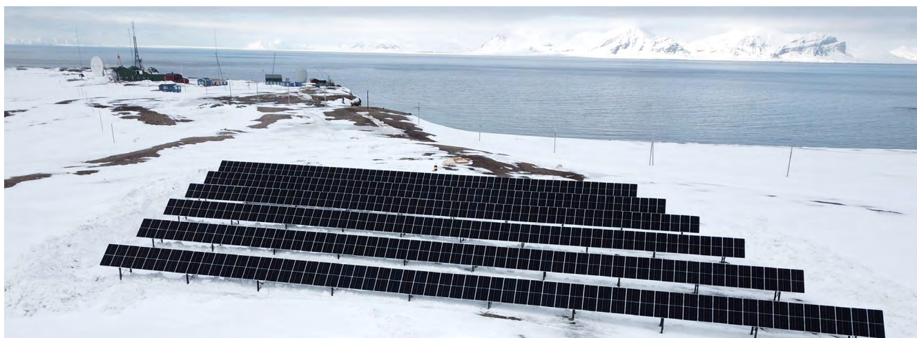
Fig. 58 - The world's northernmost ground mounted PV system at Isfjord Radio, Svalbard, 78° north. Source: Store Norske
