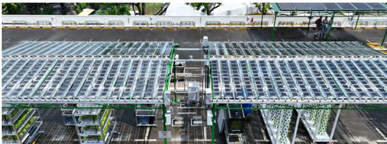
Fig. 63 - Aerial view of the Yuhua Agritech Solar (YAS) Living Lab located on the rooftop of a residential carpark in Singapore. The YAS Living Lab has 10 test-bedding projects run by institutes, companies and community members to study the combination of solar panels and urban farming for the optimum balance between crop yield and renewable energy generation on the same area. The solar roof invented by SERIS features moveable louvers that allow to track the sun during the day and are also used for rainwater management and control of the microclimate around the plants. (Image credit: SERIS).
