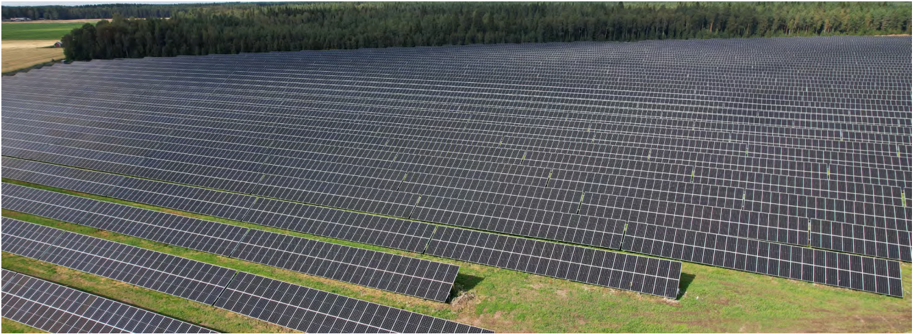
Fig. 42- Solarigo Systems Oy built Finland's largest solar power park (13 MWp) as part of the Juurakko hybrid park in Kalajoki in 2022-2023. (Photo: Solarigo Systems Oy)
