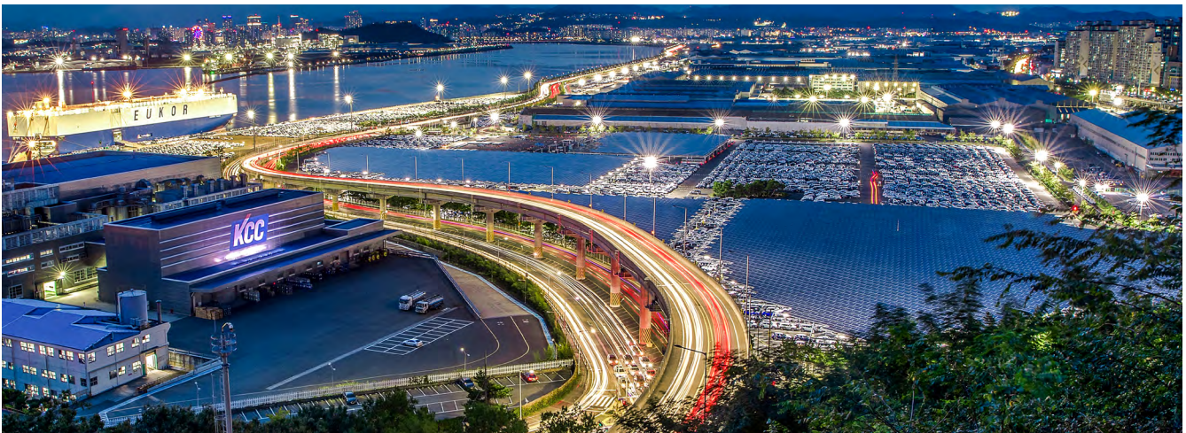
Fig. 53 - PV on vehicle loading area at Hyundai Motors, Ulsan, Korea.
