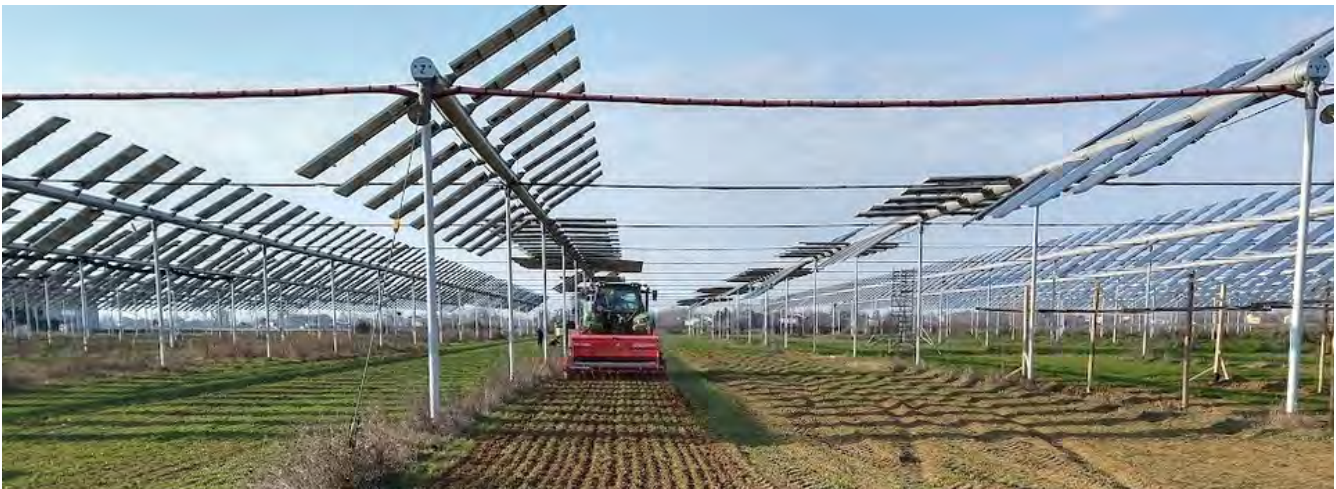
Fig. 49 - Innovative integrated solutions of agrivoltaic plant with assembly of modules elevated from the ground, Borgo Virgilio, nominal power 2,15 MW (Photo courtesy of RemTec)
