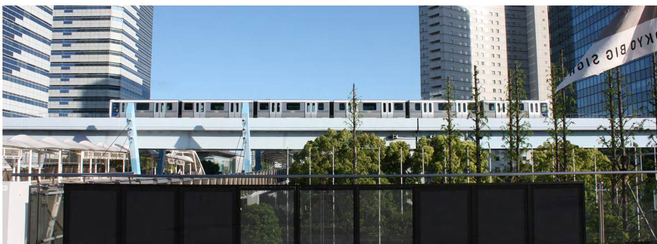
Fig. 52-PV system at Tokyo Big Sight in Koto Ward, Tokyo (T-Green® Multi Solar, building-integrated PV (BIPV) modules, see-through type and solid type, jointly developed by TAISEI and KANEKA) PV power generation capacity: 0.68 kW ©RTS Corporation
