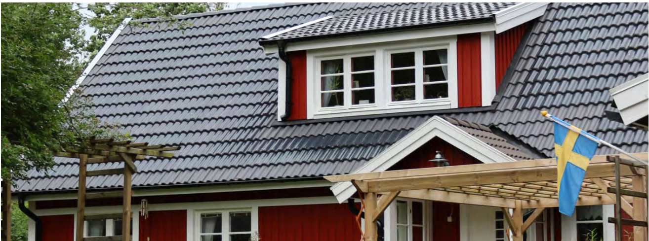
Fig. 72- Residential house with PV roof tiles produced in Sweden by Midsummer. (Industry & Market Development)
