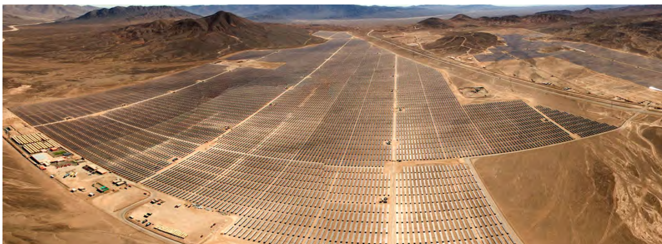
Fig. 55- The Noor Midelt complex is set to host one of the world's largest capacities for renewable solar energy and storage, boasting a total installed capacity of approximately 1600 MW. © Antonio Garcia/Unsplashq<w
