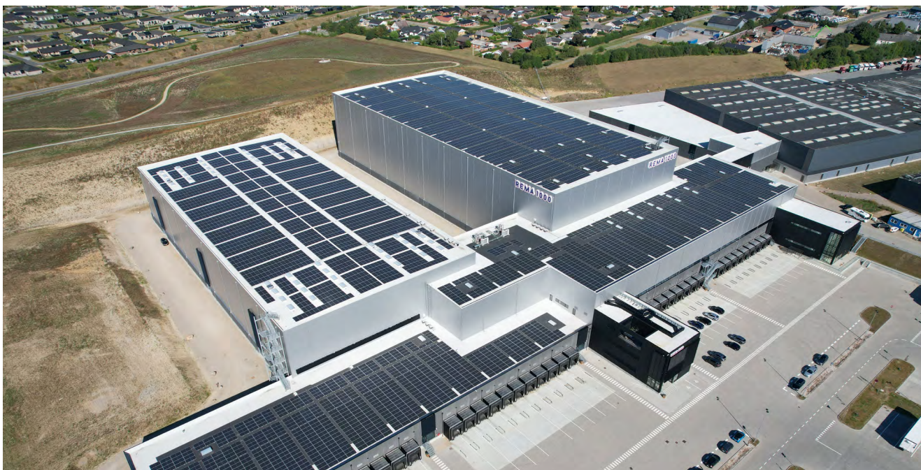
Fig. 40 - Rema 1000's new headquarters and central warehouse is one of Denmark's largest roof-based PV systems with a capacity at 3.42 MWp covering a total area of 19,000 square meters. Phønix Tag Energi A/S supplied the PV system. Photo: Amatech
