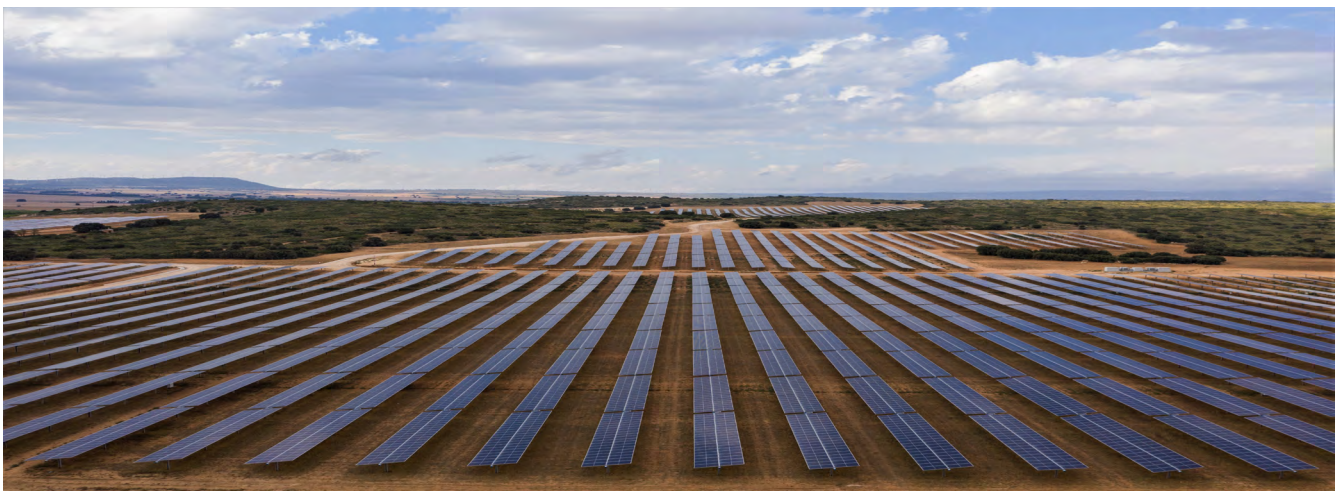
Fig. 71 - Utility-scale PV power plant. Courtesy of Solar Steel Gonvarri.
